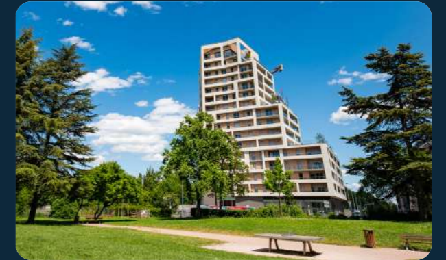
Plein Ciel • Strasbourg (67) Denu & Paradon Architecture
